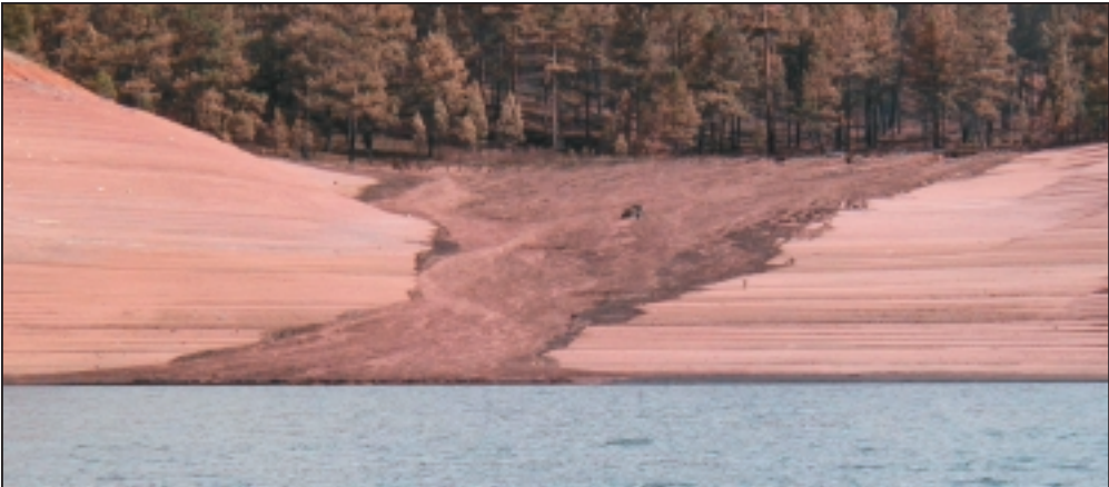
Impacted Shore. Stream bedload transported into reservoir.
