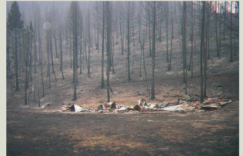
Figure 5. A structure destroyed by the Cave Gulch fire, part of the Canyon Ferry complex.
