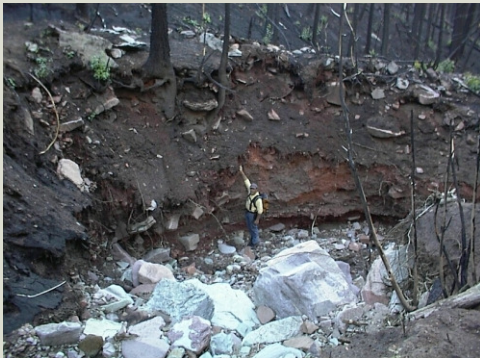
Figure 15. Serious erosion after the Missionary Ridge fire damaged water quality, flow regimes and aquatic habitat. (Image credit: Larry Woodson)
