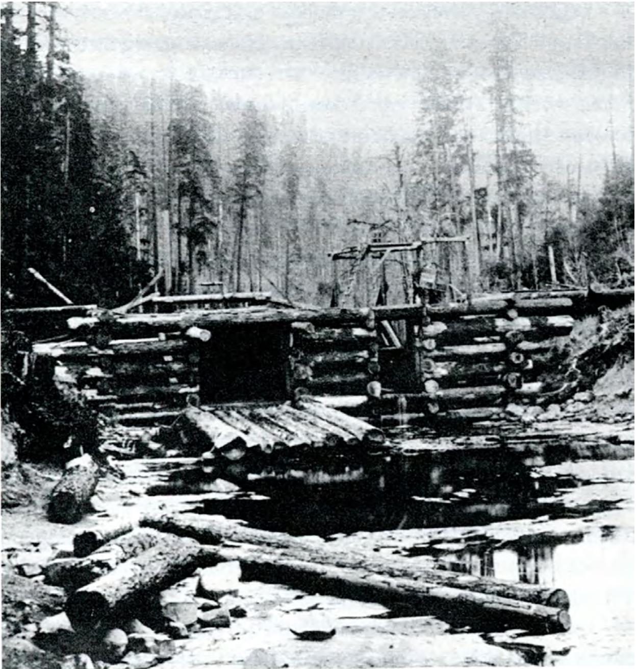
*Above. Constructed of log cribs, this self-tripping dam on Mill Creek spanned the stream deep in the forest. Opposite. Workmen for the Gardiner Mill Company constructed a series of crib splash dams on Mill Creek near Loon Lake in the lower Umpqua River region.*
