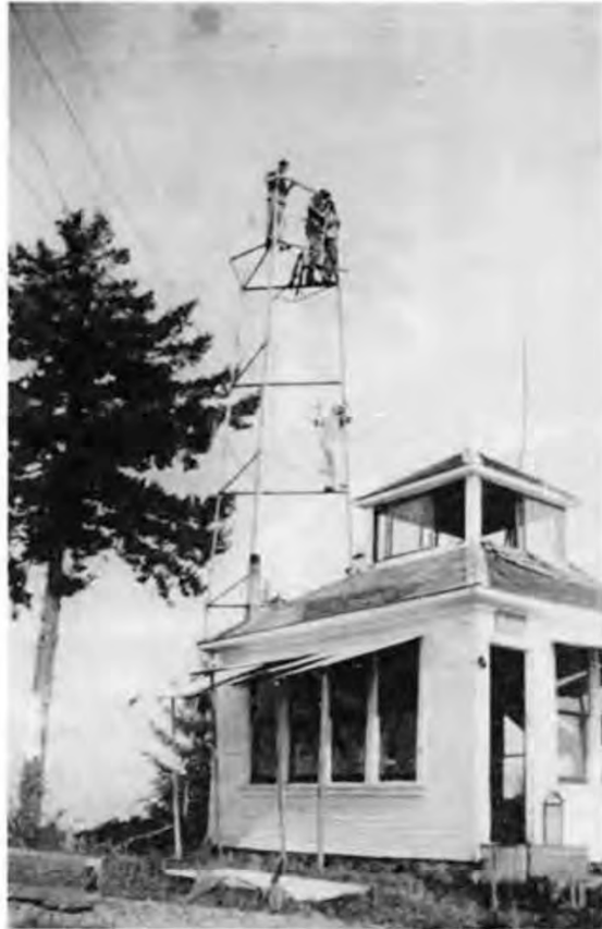
Between August of 1939 and July of 1940, CCCs built a 20-foot lookout tower, a 3-room cabin, and a woodshed on Dean's Mountain. It's interesting to wonder what today's safety standards would call for in the work shown here. —Photo courtesy of Inez Miller, Bandon.
