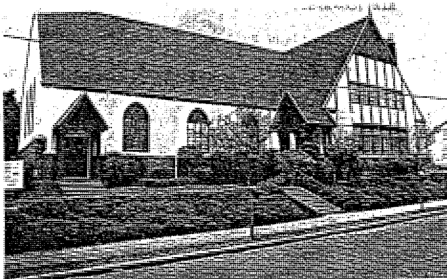
4635 NE 9th Avenue. Highland Congregational Church, 1926.
