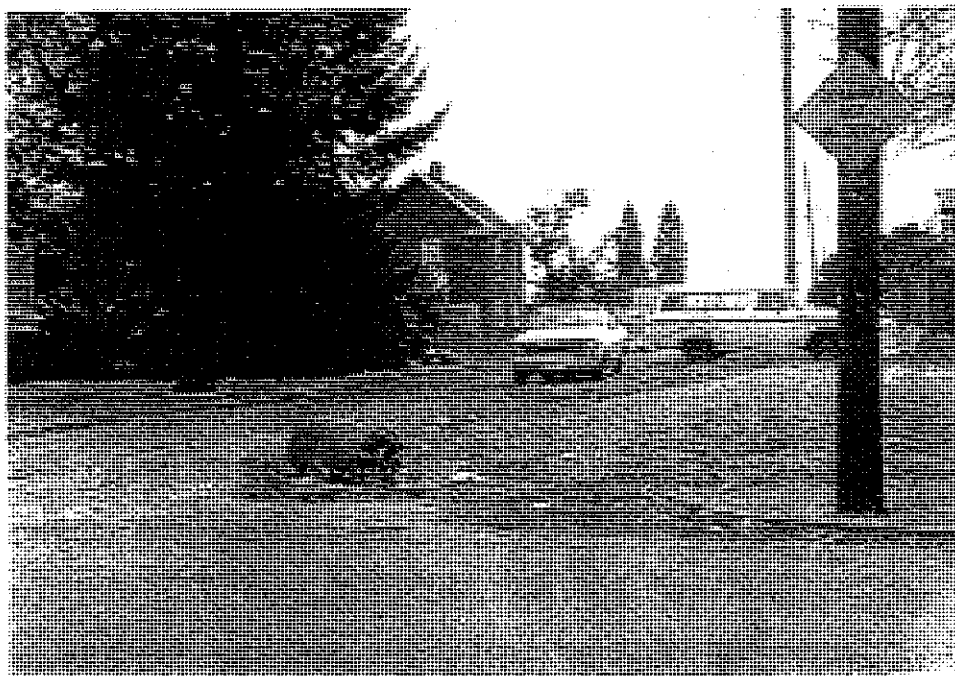
Fig. 76 Unpaved Streets: 24th & Wygant (T. Ward)
