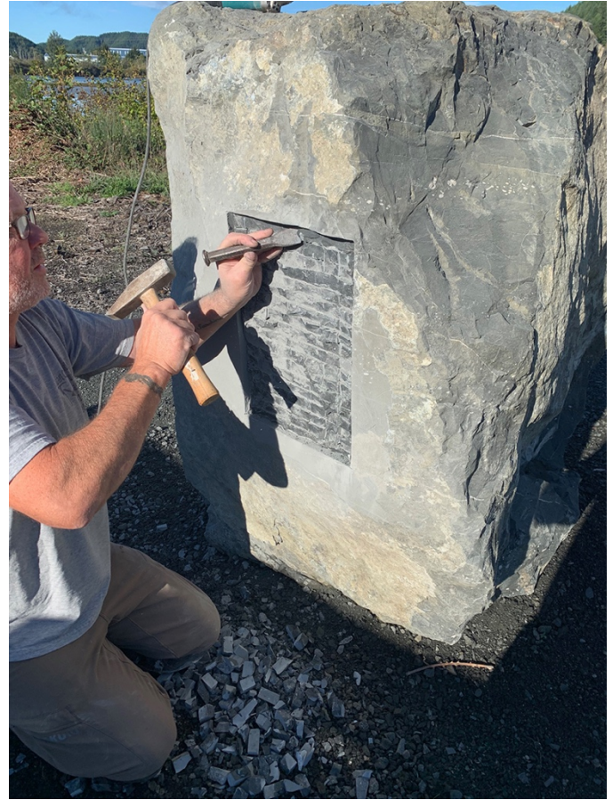
(L) Stu Richardson, Richardson Masonry, Reedsport, Oregon, cutting patterns into Umpqua Memorial Stone with diamond grinding wheel to house bronze plaque. (R) Stu chiseling sections from stone made by grinding wheel. Photos by Richardson Masonry apprentice, Jason Richer, October 15, 2023.
