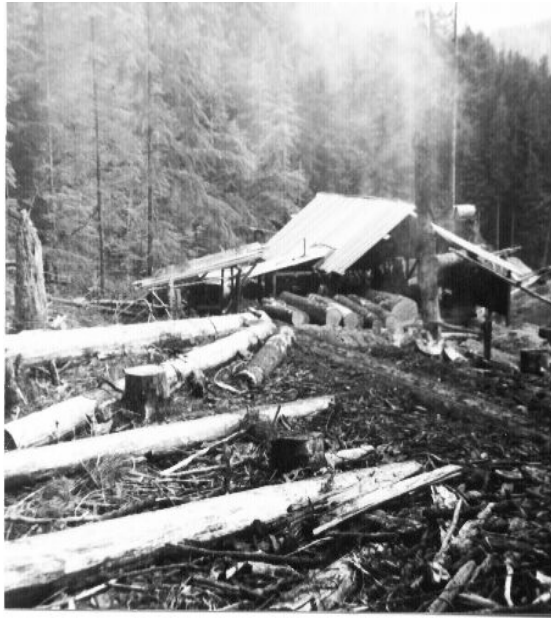
The completed mill, June, 1940, set in the timber at top of a hill with no road to it.
