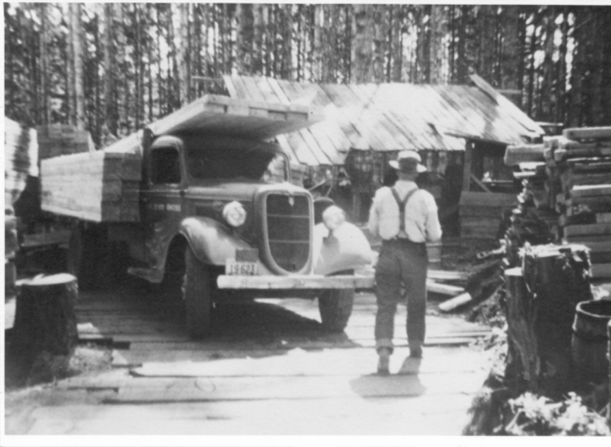
George Youst's first sawmill in Coos County, 1937. Located near Hauser, it is set "in the woods." Note the 65-year-old Douglas fir timber still standing behind the mill and the stumps on each side of the plank road. The truckload of lumber, ready to go to town, contains 100 16 ft 2x10's and 12 24 ft 2x10's – about 3,100 board feet of lumber. This mill might put out three such truckloads, on a good day.
