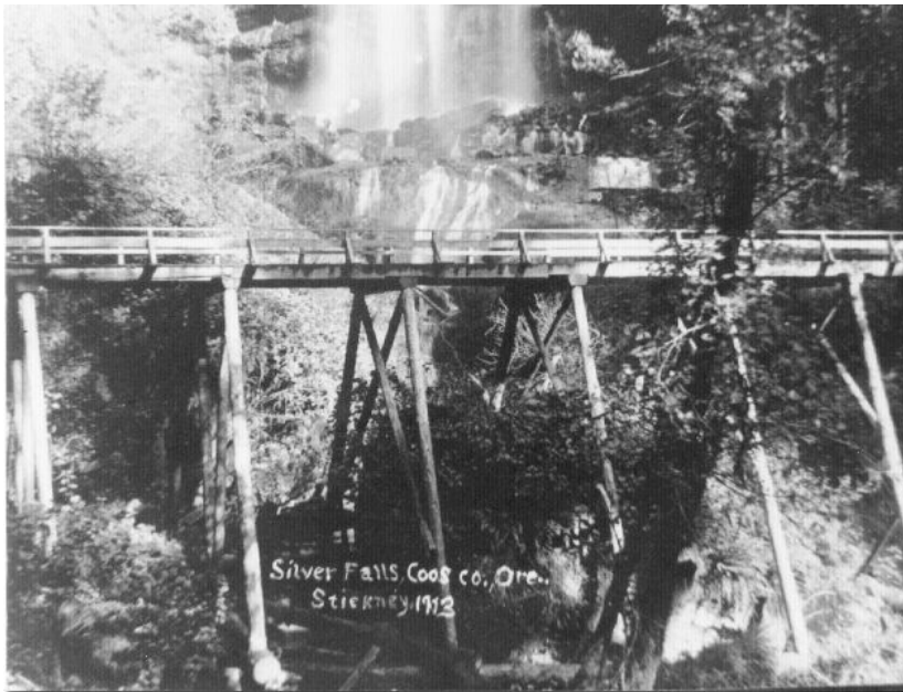
The Silver Creek Bridge, built in 1909. In 1943 the first two bents of the bridge – far right – were rotten and collapsed with a truck load of lumber from Dad's mill. He brought the mill crew down, cut logs to replace the rotten posts, cut plank at the mill for the stingers and deck, and put the bridge back into service in a few days. That repair was still good in 1958 when the county finally removed the bridge and closed the road for good.
