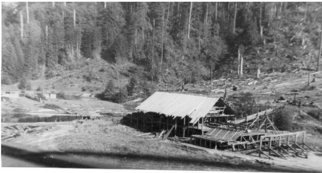
The mill in its second setting. The mill pond with logs in it, left. The dam in Glenn Creek was behind the mill. This picture was taken before the roof had been extended over the loading docks, right. This mill averaged about 20 thousand board feet of dimensioned lumber per day through most of World War II.
