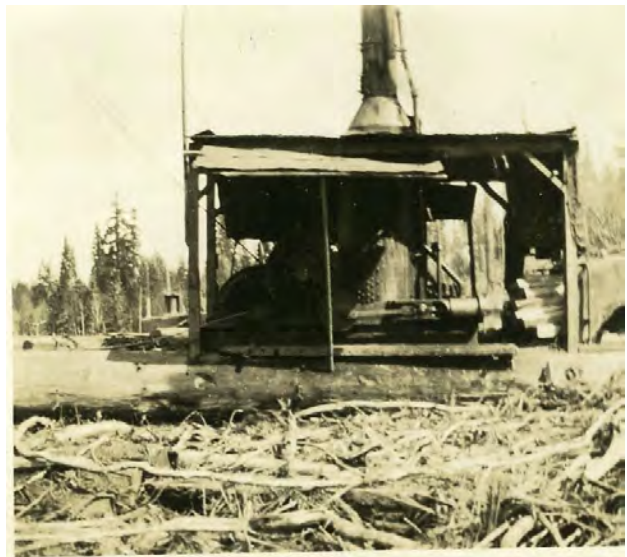
George Youst's 10 x 12 Seattle steam donkey with the new sled he built for it.
