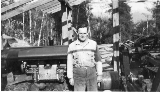
Dad standing in front of the GMC diesel power unit. He had two of those engines to run the mill – one to run the headrig and feedworks, the other ran the edger, trim saws, and conveyors.
