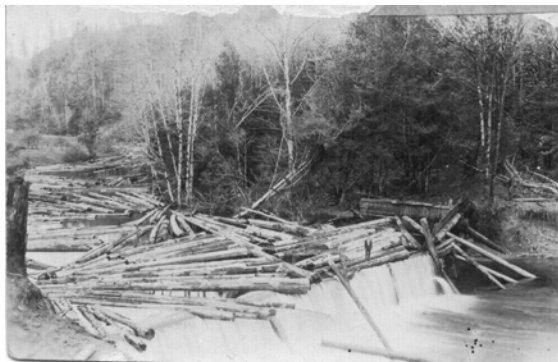
Splash dam on Millicoma River West Fork, after a freshet had brought logs down on top of it.
