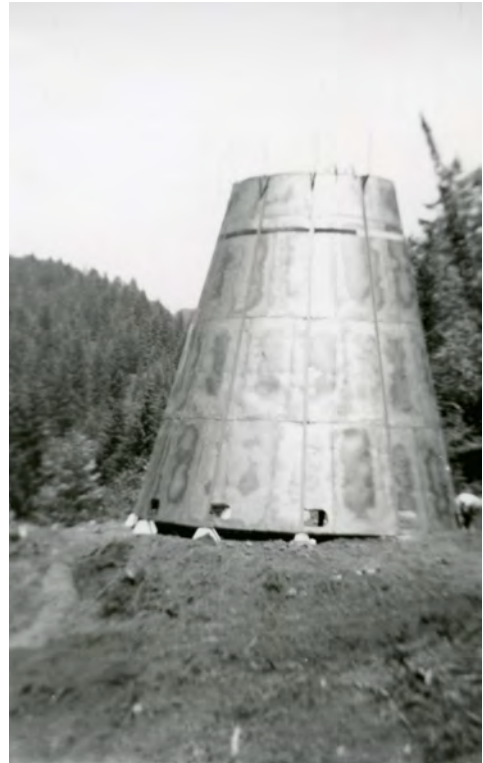
Dad's first wigwam burner being assembled at the Ash place near Allegany, Oregon, 1953.
