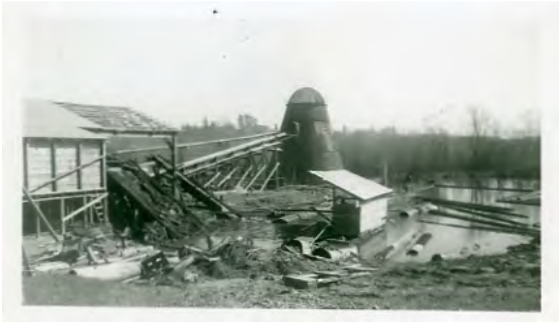
George Youst sawmill, Forestville, California, 1955. This was an all-electric mill, with a planer, and 8-hour capacity of 30,000 bd. ft.
