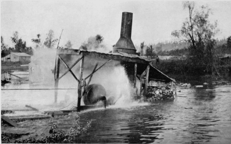
Emerging on the opposite bank. Steam pressure 75 pounds.
