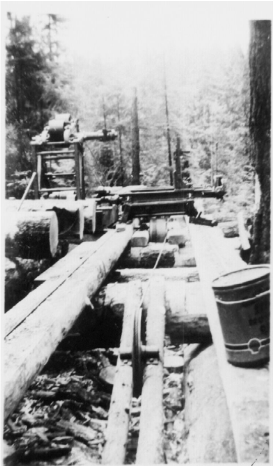
Mill under construction, showing carriage tracks, saw husk, and part of log rollway. Dad hand hewed the carriage track stringers from logs.
