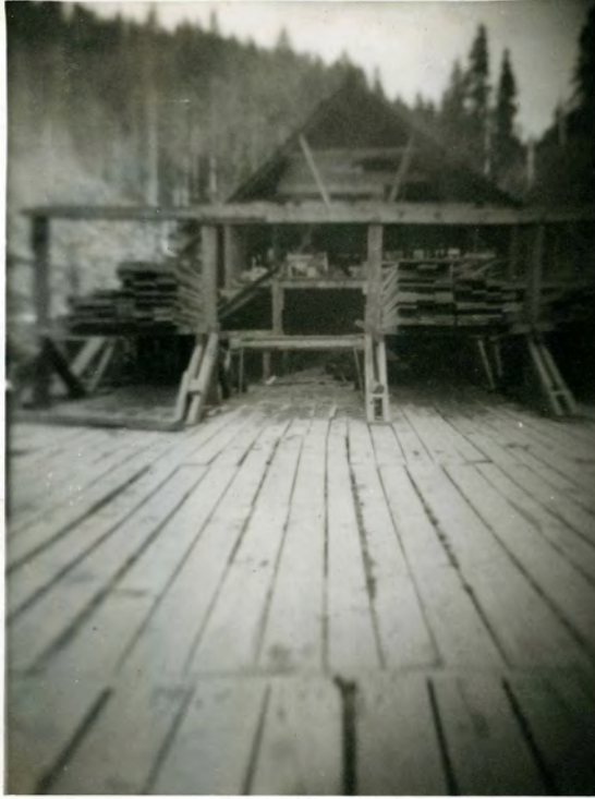
The loading dock area of the mill, showing loading jacks. The trucks would back under the loading jack, which is pre-loaded with 4,000 board feet of lumber ready to go to town.
