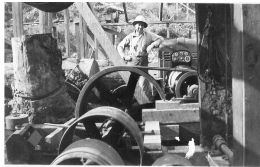
Inside the mill, under construction. Dad standing alongside of the GMC diesel power unit. Note the notched guyline stump inside the mill!
