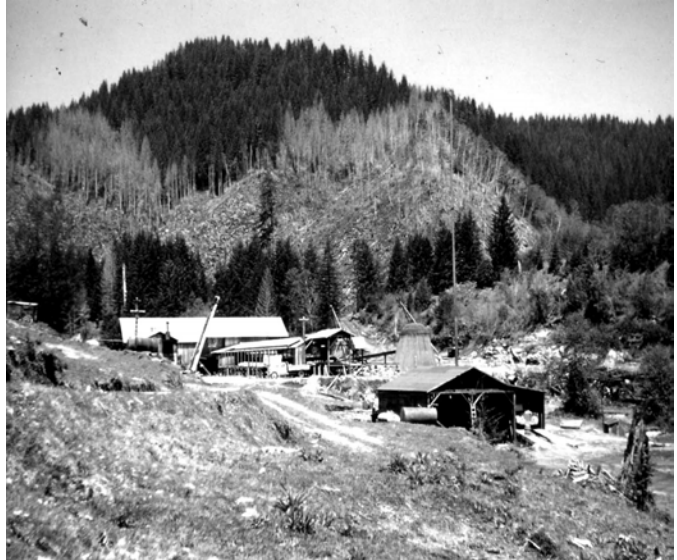
George Vaughn sawmill on private land adjacent to the Elliott State Forest, 1955. The green timber in the background is State land.
