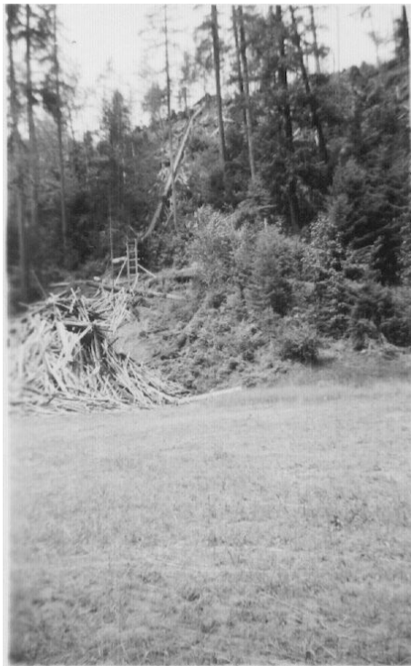
Slab pile with slab chute coming down from the mill at the top of the hill. The lumber chute was several hundred feet further down the field, to the left.
