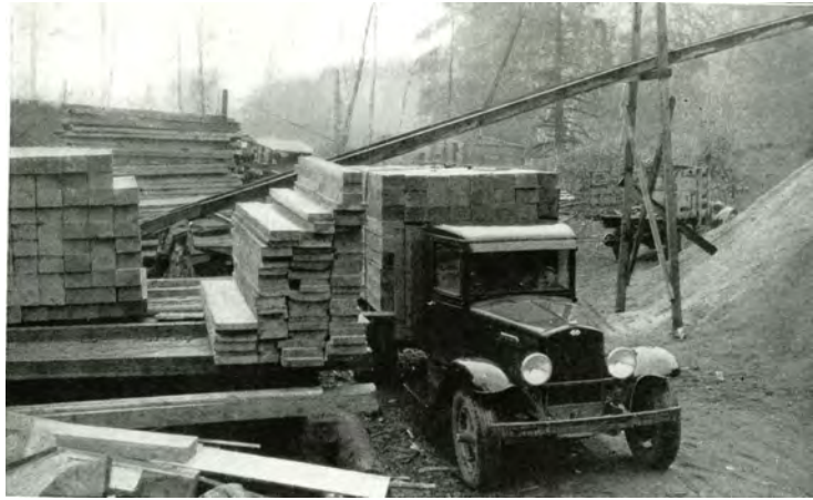
Back end of a typical tie mill of the period, 1920's and 30's. Note sawdust conveyor and sawdust pile at right. At left, stack of ties and 2-inch side cut. From Timberman, May, 1934, p. 16.
