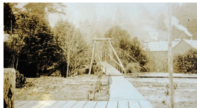
Walking bridge between the barracks and main camp buildings across the Middle Fork of the Coquille River. The kitchen and part of the mess hall can be seen on the right; ca. 1934. Photo courtesy of the Oregon Historical Museum album.
