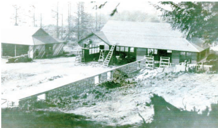
The enrollees from the Gold Beach Camp are seen here building the USFS Gold Beach Ranger Station. Note the fine rockwork. The ranger station was put on the National Registry of Historic Buildings on April 8, 1986. Photo courtesy of the U.S. Forest Service Ranger Station at Gold Beach, Oregon.
