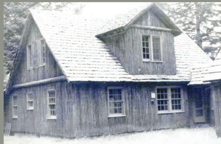
The Cedar House was all that was left when in 1979 Dr. Stephen Dow Beckham conducted an inventory of all the CCC camps in the Siskiyou National Forest. This is the west-facing view of the Cedar House. Photo courtesy of Dr. Stephen Beckham.
