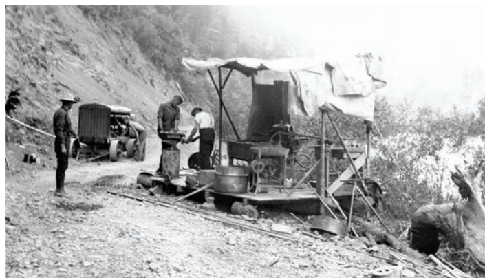
A blacksmith came right to the job site on the Agness-Gold Beach roadway to fabricate material for the construction work; ca. 1935. Photo courtesy of the U.S. Forest Service Ranger Station at Gold Beach, Oregon.
