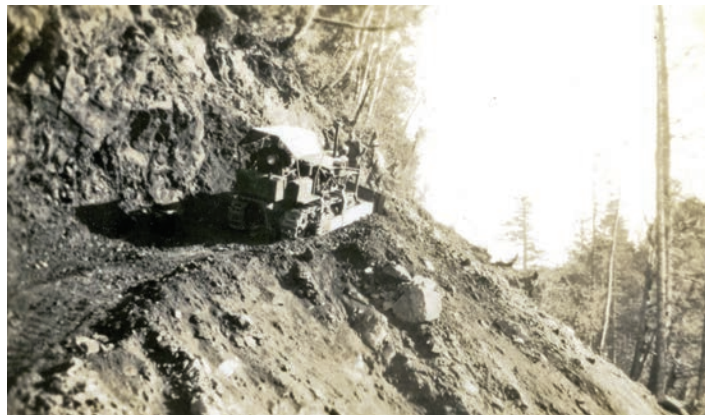
The Cletrac tractor building a roadway near Agness, Oregon ca., 1933. Photo courtesy of Ms. Alice DeSoto.
