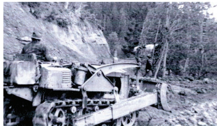
The CCC Cletrac bulldozer seen here building the roadway near the Agness Pass on the way to Powers, ca. 1935. Photo courtesy of the U.S. Forest Service Ranger Station at Gold Beach, Oregon.
