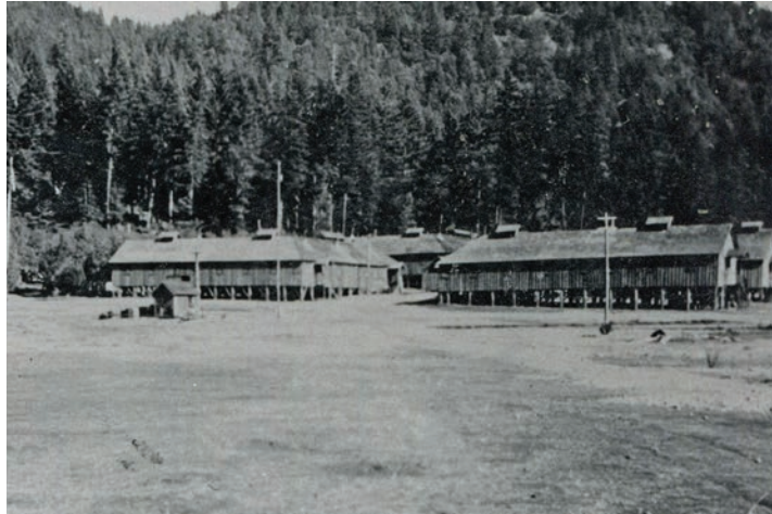
Agness Camp; ca. 1937. Several of the boys at the camp in '38 were from the towns of Myrtle Point and Powers. 105 Photo courtesy of the U.S. Forest Service Ranger Station at Gold Beach, Oregon.
