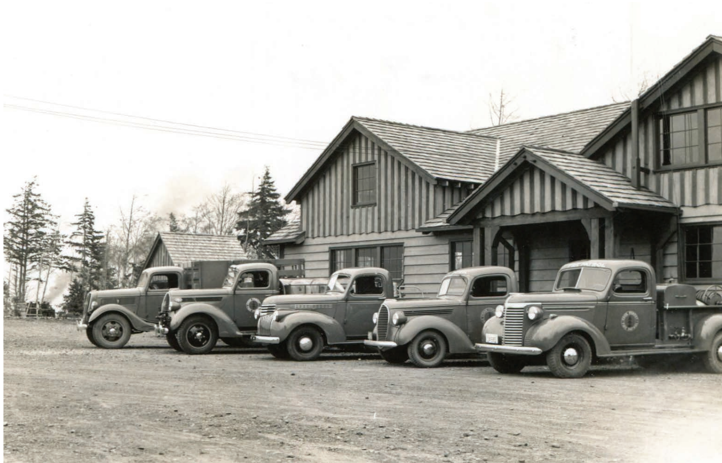
Top: Coos Forest Protective Association headquarters, built by the CCC. Bottom left: Entrance sign to the Coos Forest Protective Association headquarters on Bunker Hill. Bottom right: Residence at the Coos Forest Protective Association headquarters. The headquarters building of the Coos Forest Protective Association was built by Company # 981 as a side camp from Camp Walker in 1936–37. In the first year, they built a warehouse, a 60-foot lookout tower, the main office building, and a residence. Photos courtesy of the Coos Forest Protective Association, Coos Bay, Oregon.
