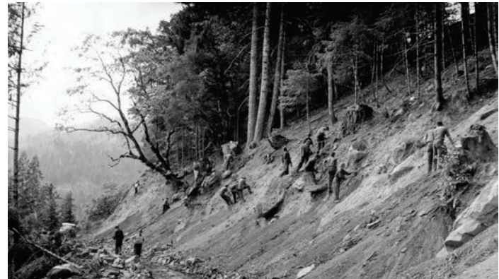
The above photos show the CCC boys from China Flats Camp sloping the road bank on the road from Powers to Agness, ca. 1935. Photo courtesy of the U.S. Forest Service Ranger Station at Gold Beach, Oregon.
