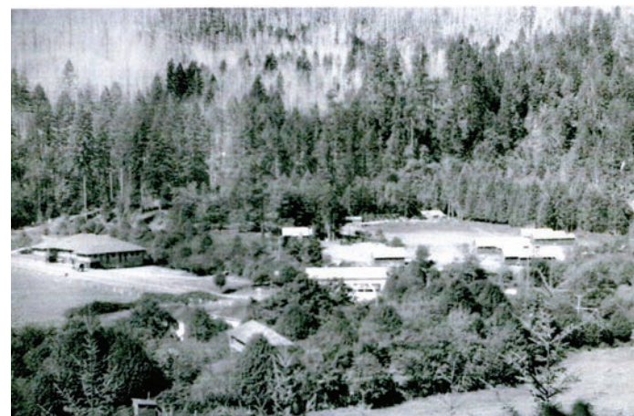
Bird's eye view of Camp Bradford; ca 1934-35. Note the large resort/barracks structure at the left side of the photo. The road between Myrtle Point and Roseburg runs just in front of the lodge building. Photo courtesy of the NARA.
