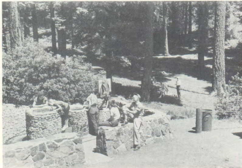
Tub Springs Wayside—Showing spring outlet and picnic area.
