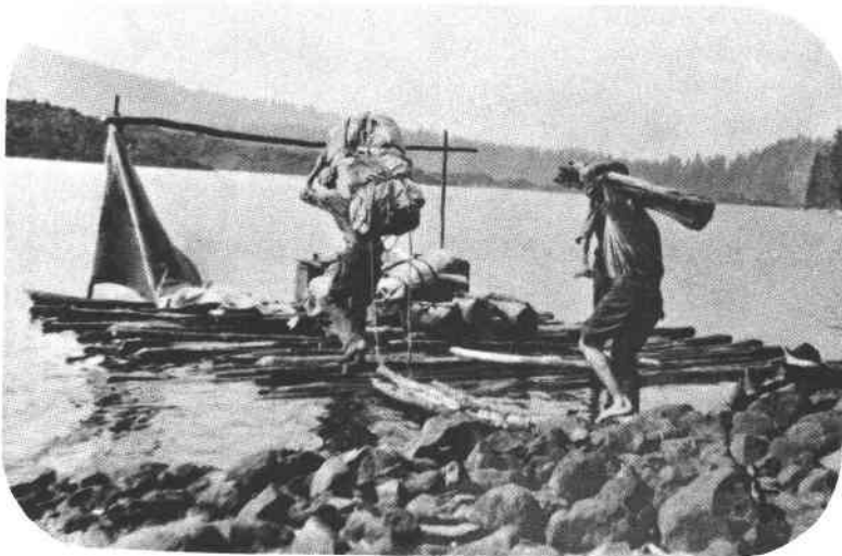
When trucks or mules could not pack in the equipment and supplies, the men had to fashion water transportation. This photo was taken about 1923.
