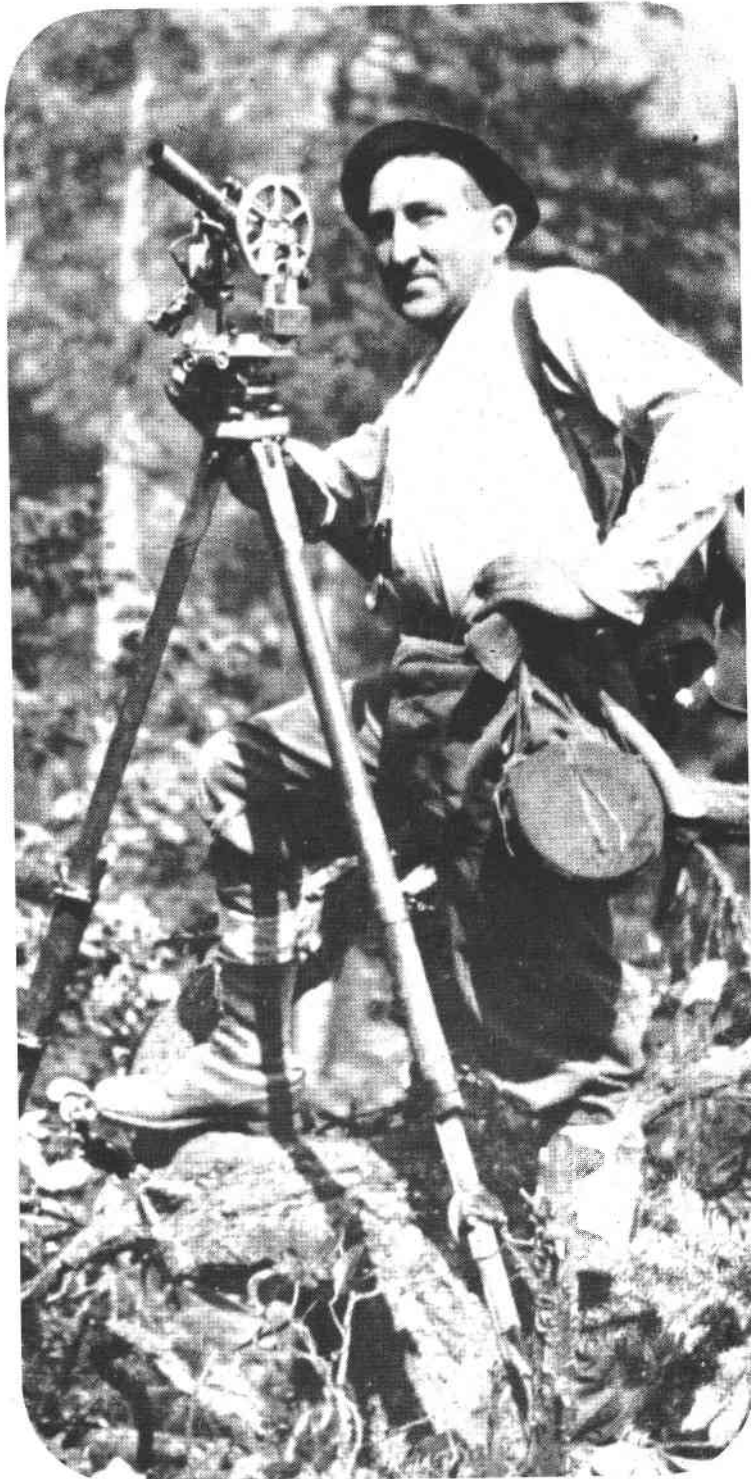
Quintin Campbell, U.S. transitman, in Oregon, 1917. The instrument is a Buff transit.
